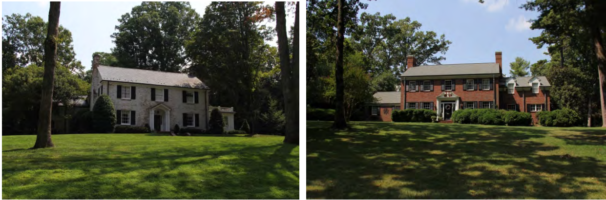
The Pines (CT1468), house at 860 8 th Street NW (l) and house at 843 7 th Street NW (r)
