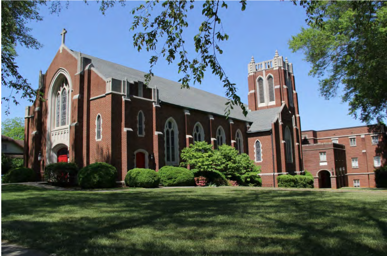
St. Andrew's Lutheran Church (CT1368), 629 8 th Street NE
