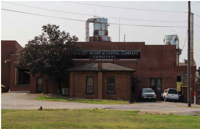
Hickory Manufacturing Company (CT1422), 9 Lenoir Rhyne Boulevard SE
