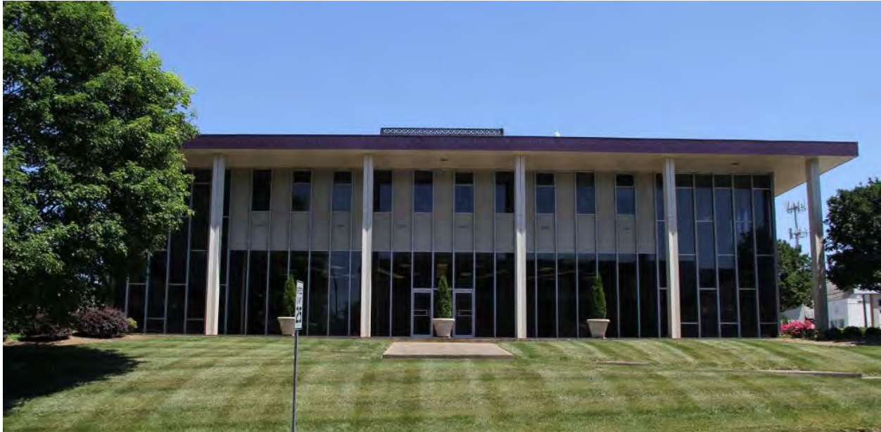
Fidelity Federal Savings & Loan Association Building (CT1382), 110 N. Center Street
