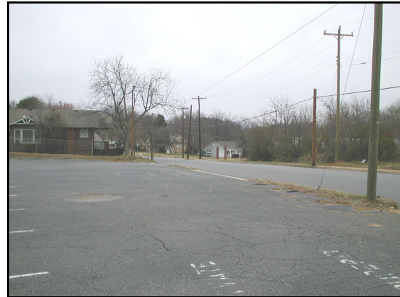
Vast parking lots and lack of landscaping contribute to the run down appearance of Highland Avenue NE.
