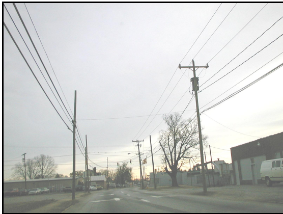
Highland Avenue NE is cluttered with numerous overhead utility lines.
