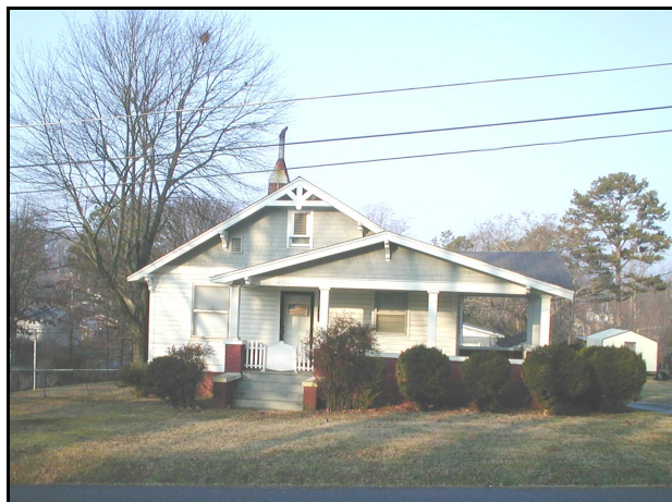
Bungalows, such as this one on 14 th Street NE, are typical of the homes found in Highland neighborhood.
