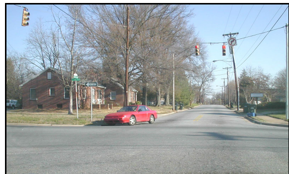
This vehicle is caught running the red light, maybe because the stop bar on the pavement is faded away, and the motorist does not know to wait behind it to trip the signal to change.
