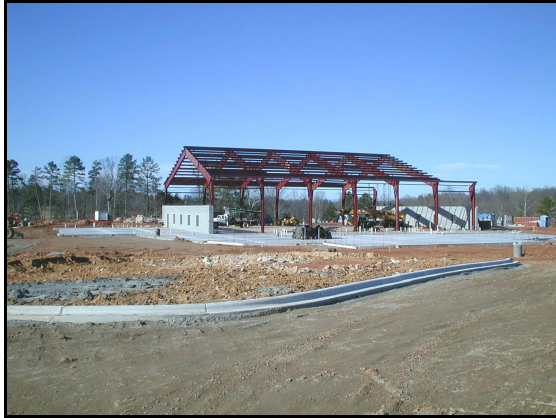
Construction on the new recreation building began in the fall of 2001.
